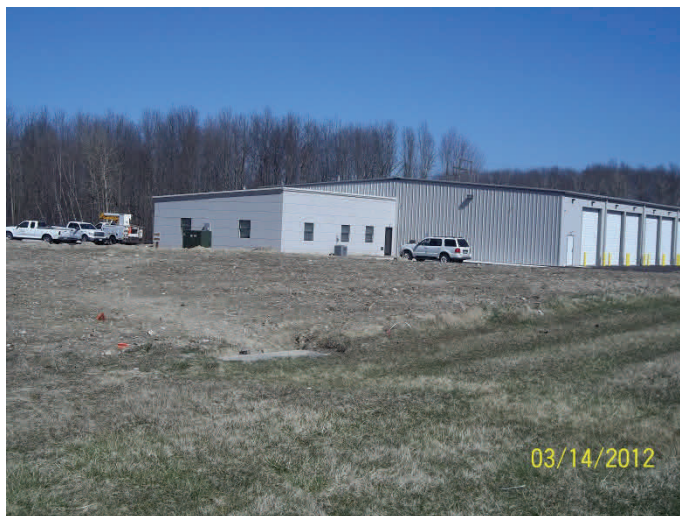
Main Lite Electric Building on Sferra Ave. NW
