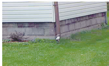
IMPROPER DOWNSPOUT
