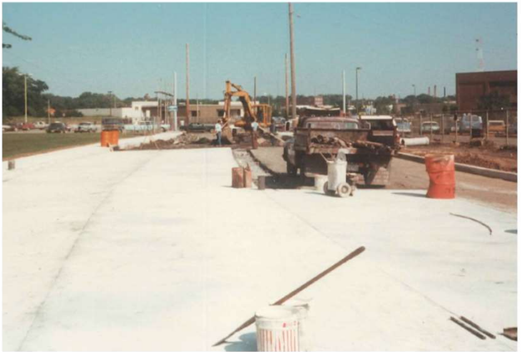
Pine Ave Widening & Storm - 1984
