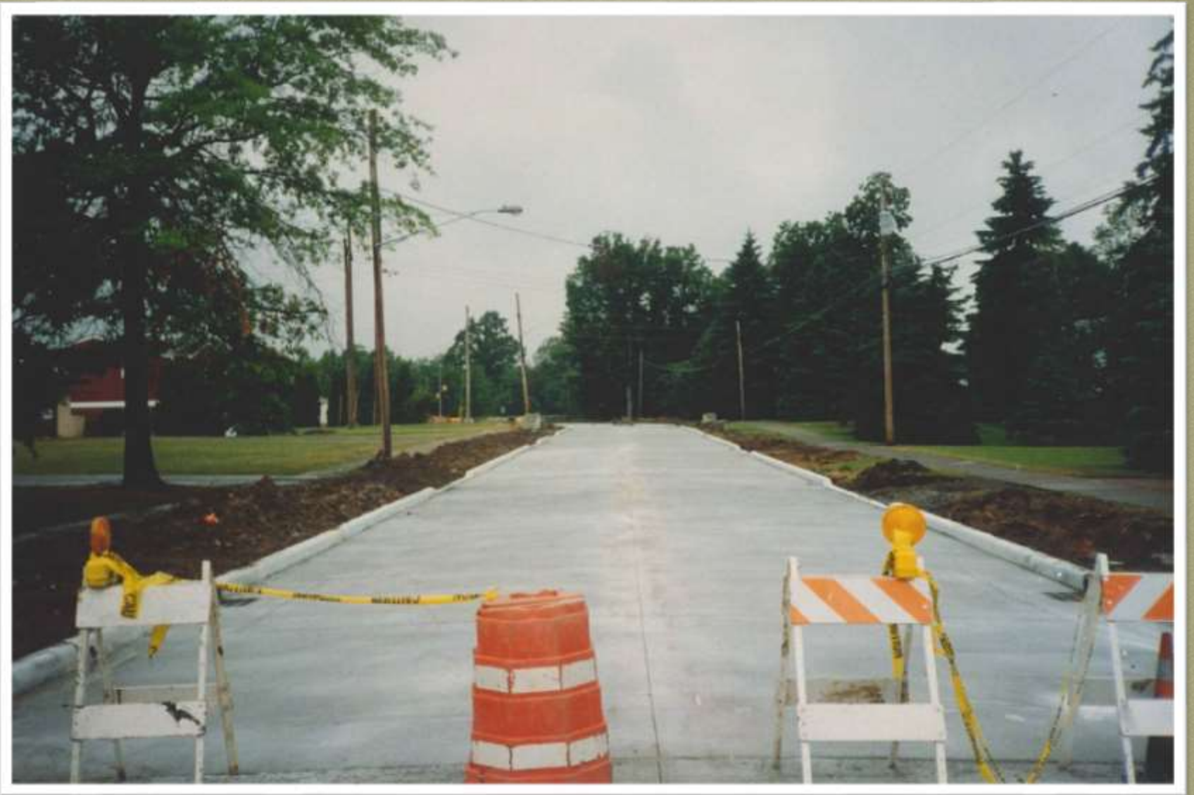
Tod Ave NW Reconstruction & Safety - 1993
