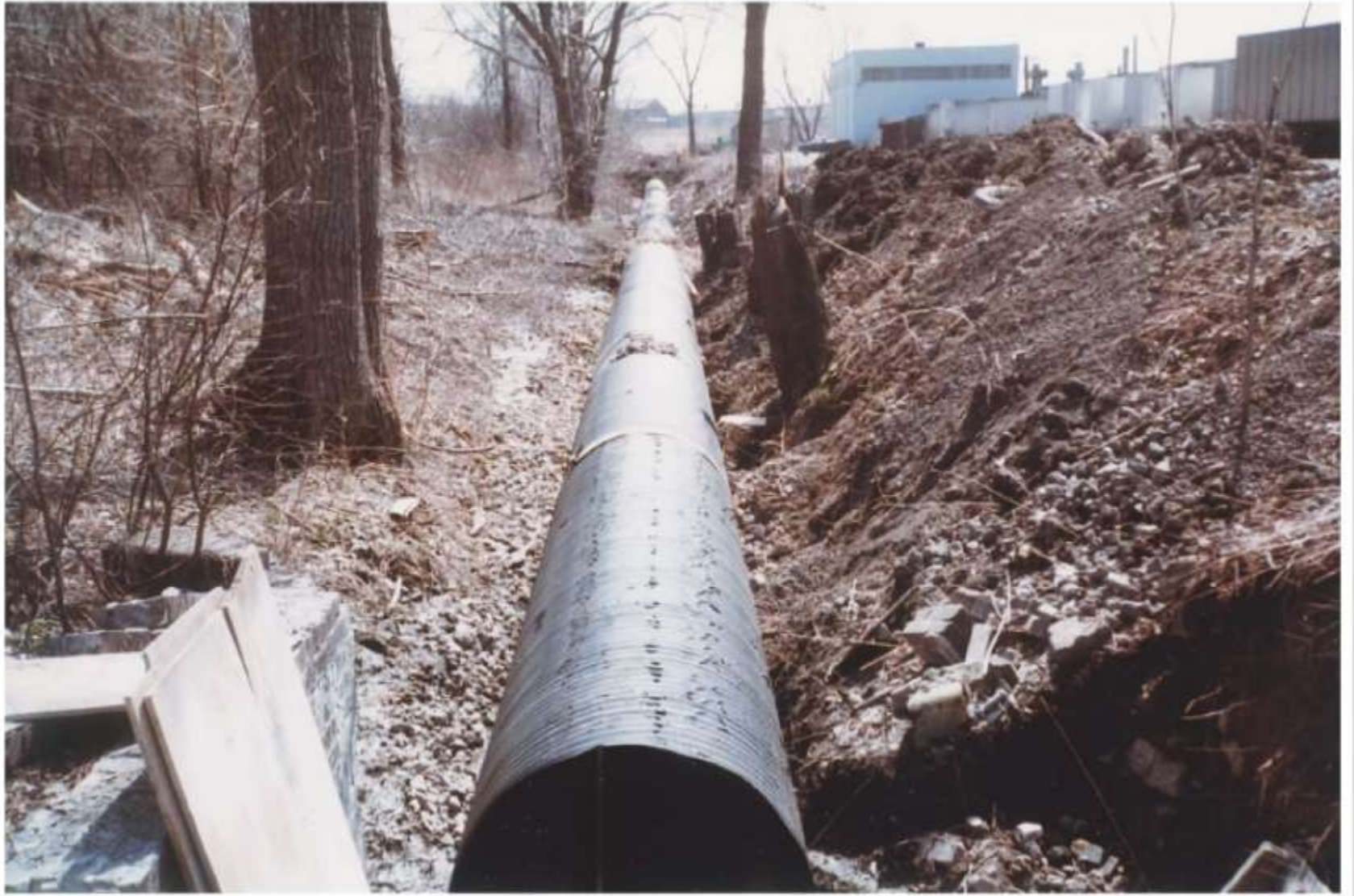
Pine Ave Widening & Storm - 1984
