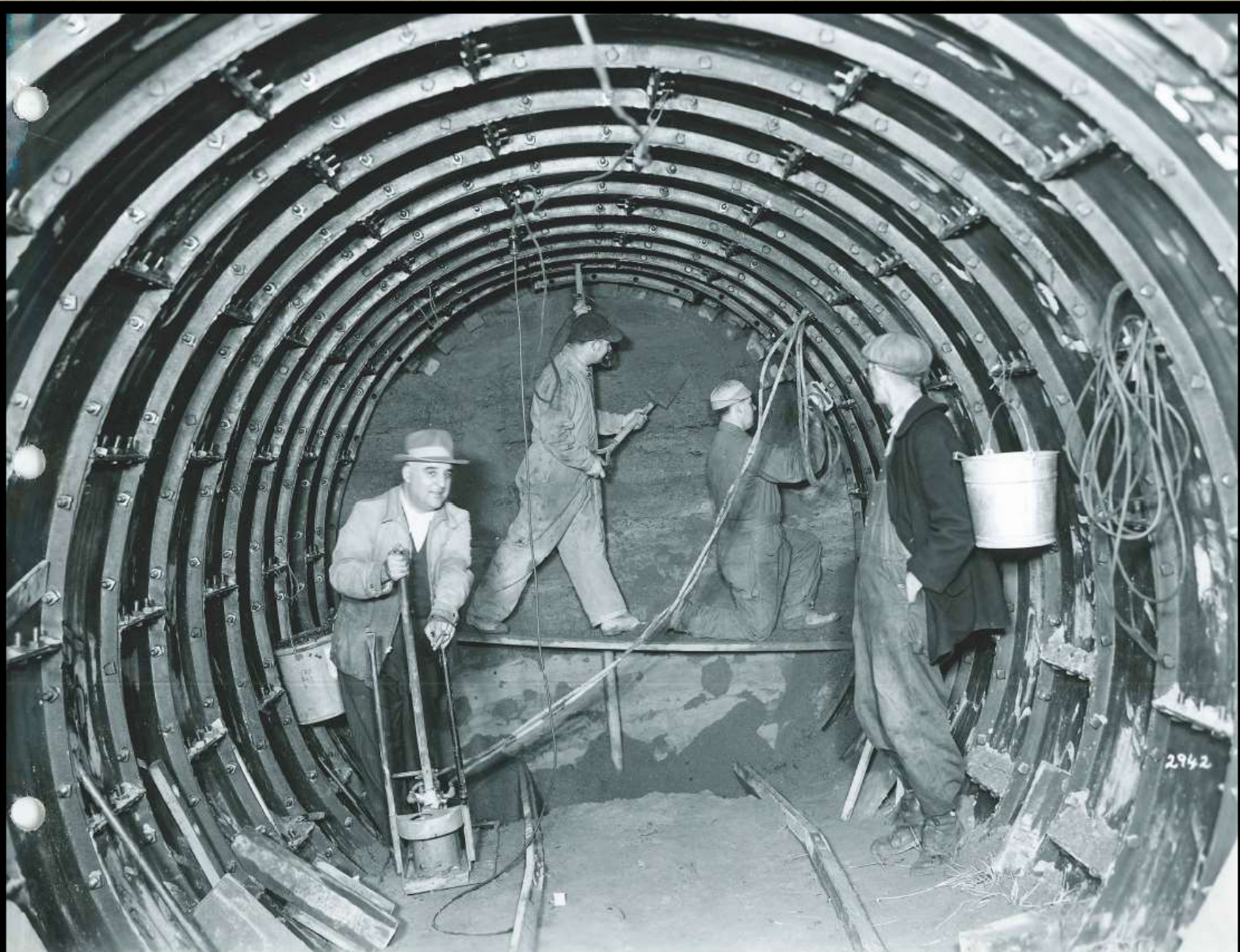
Red Run Combined Sewer (West Branch)-Tunnel Under Erie R.R.(Mainline)- Nov. 1948
