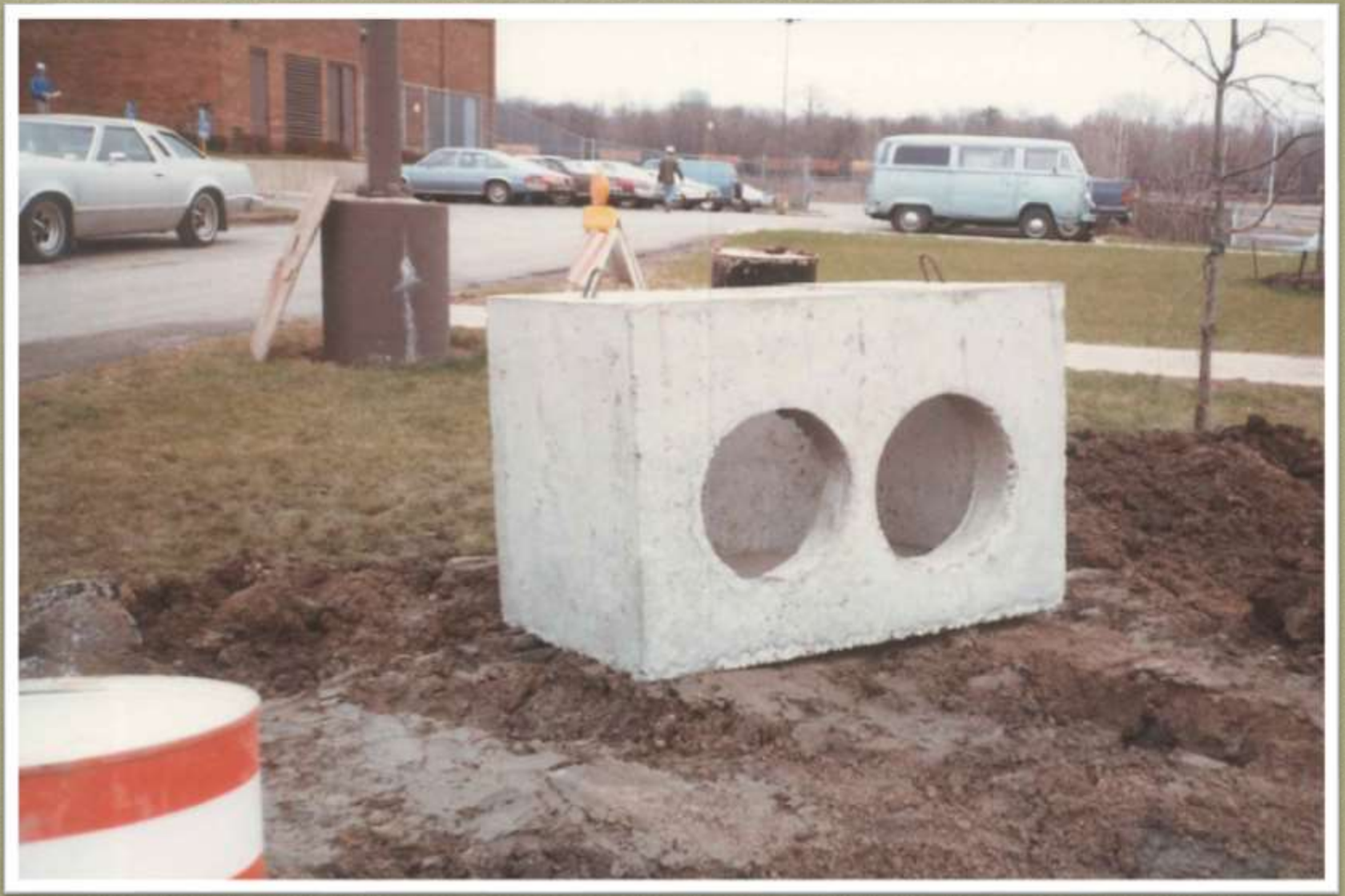
Pine Ave Widening & Storm - 1984
