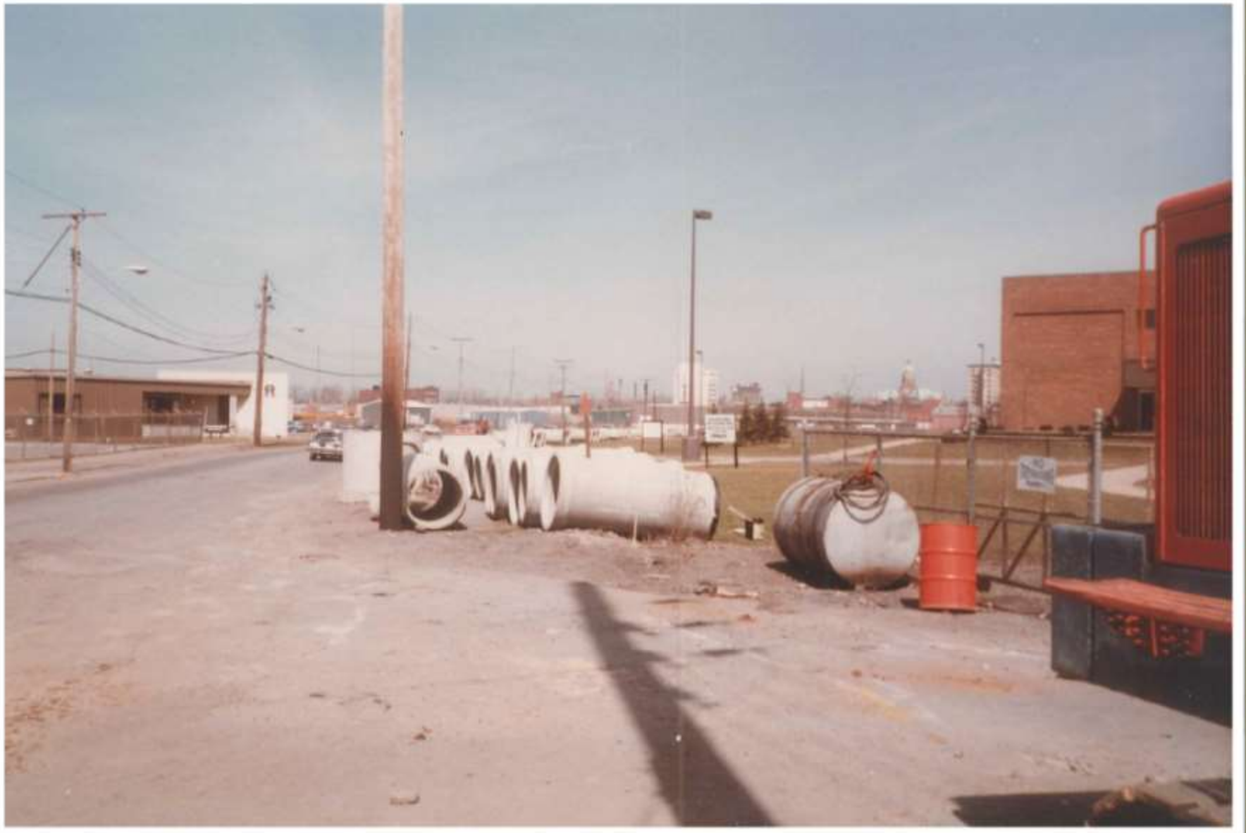
Pine Ave SE Widening & Storm Sewer - 1984
