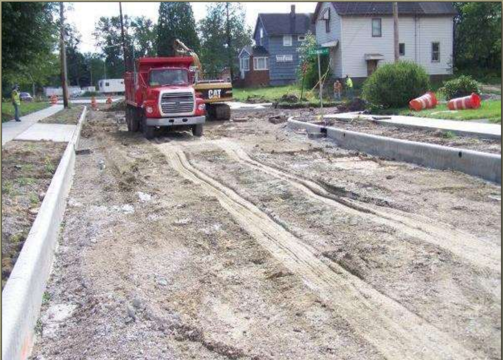
Willard Ave SE Reconstruction - September 15, 2008
