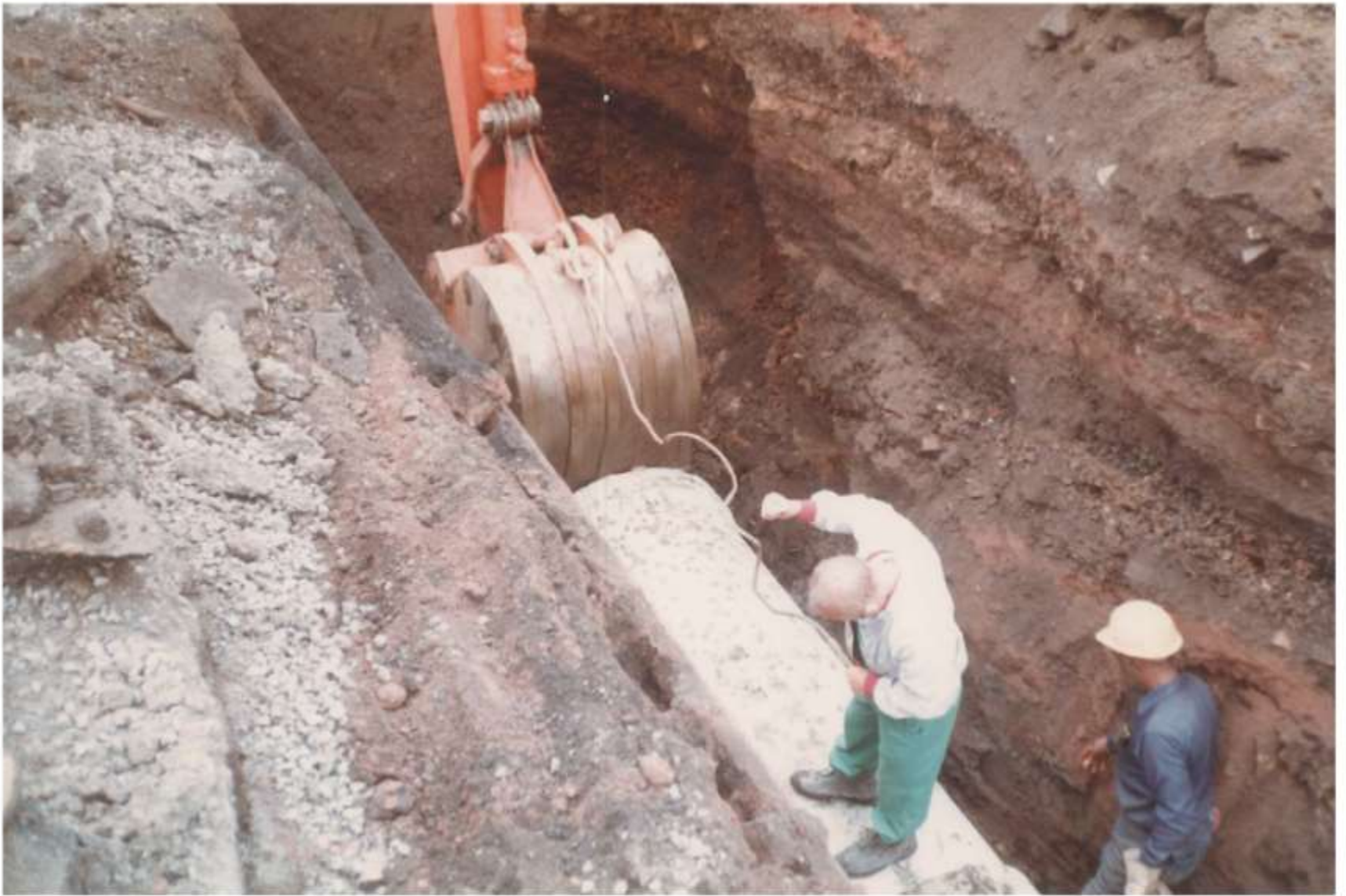
Pine Ave Widening & Storm - 1984
