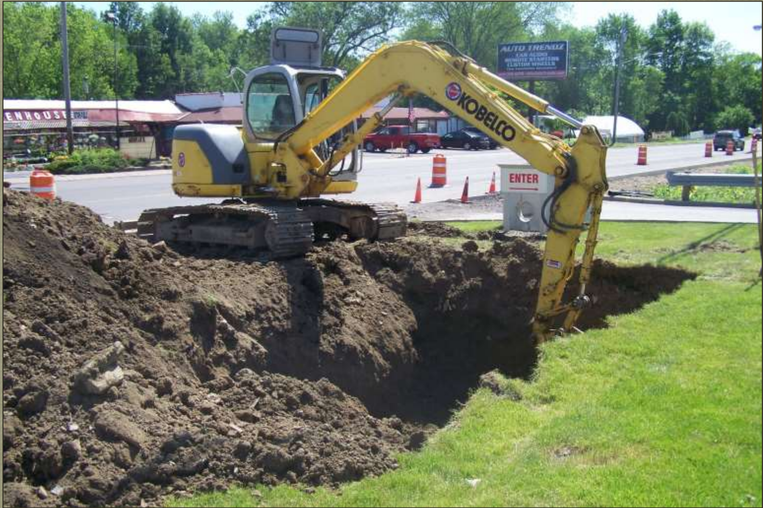
Parkman Road NW Phase 2 - 2011
