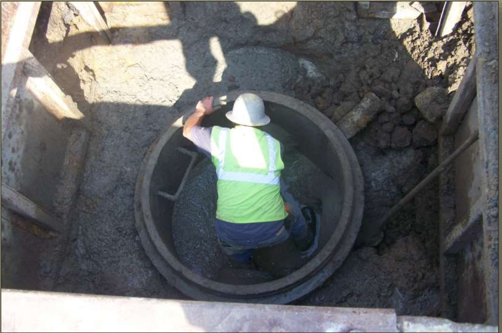
Parkman Road NW Phase 2 - 2011
