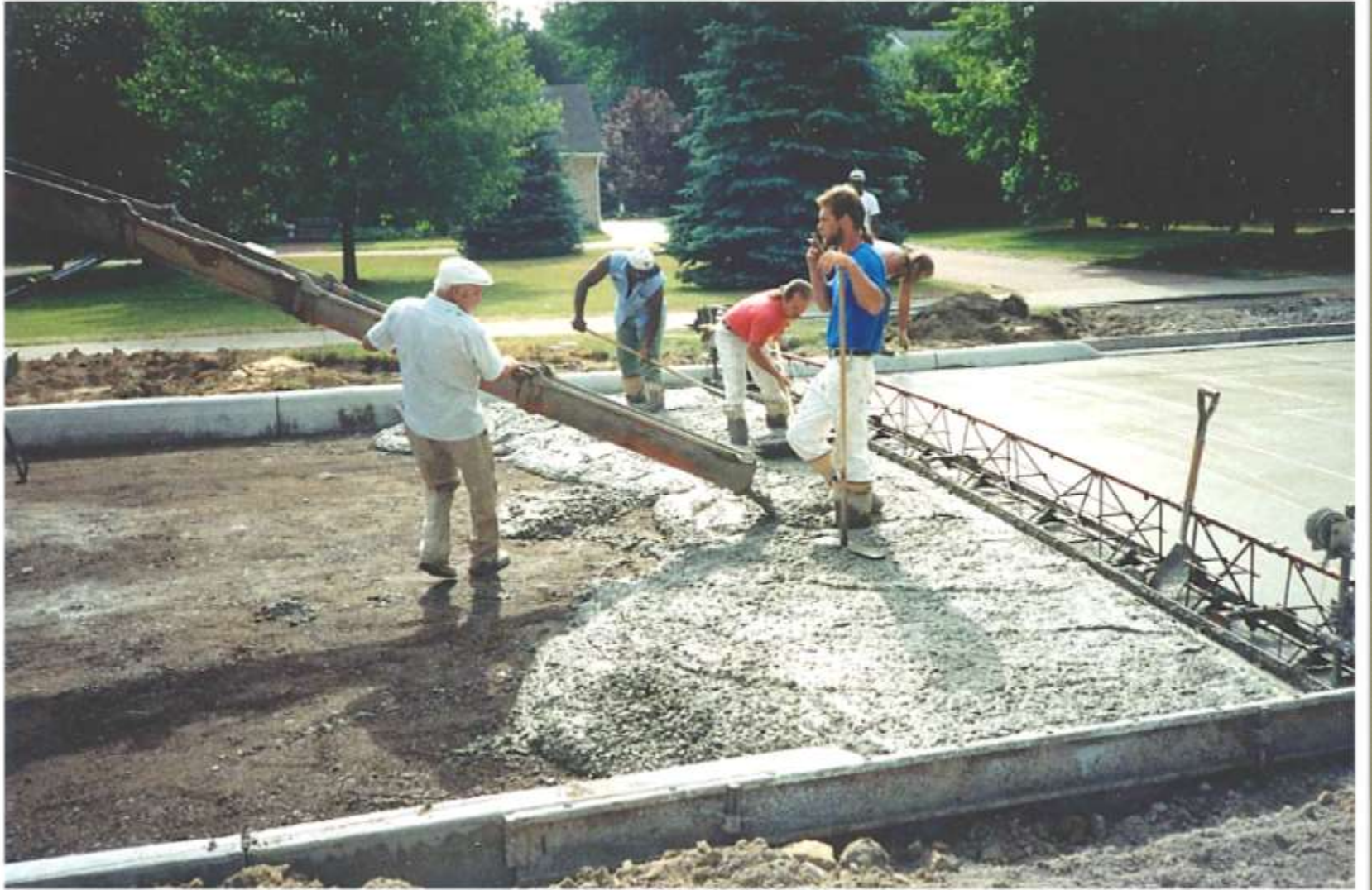
Tod Ave NW Reconstruction & Safety - 1993
