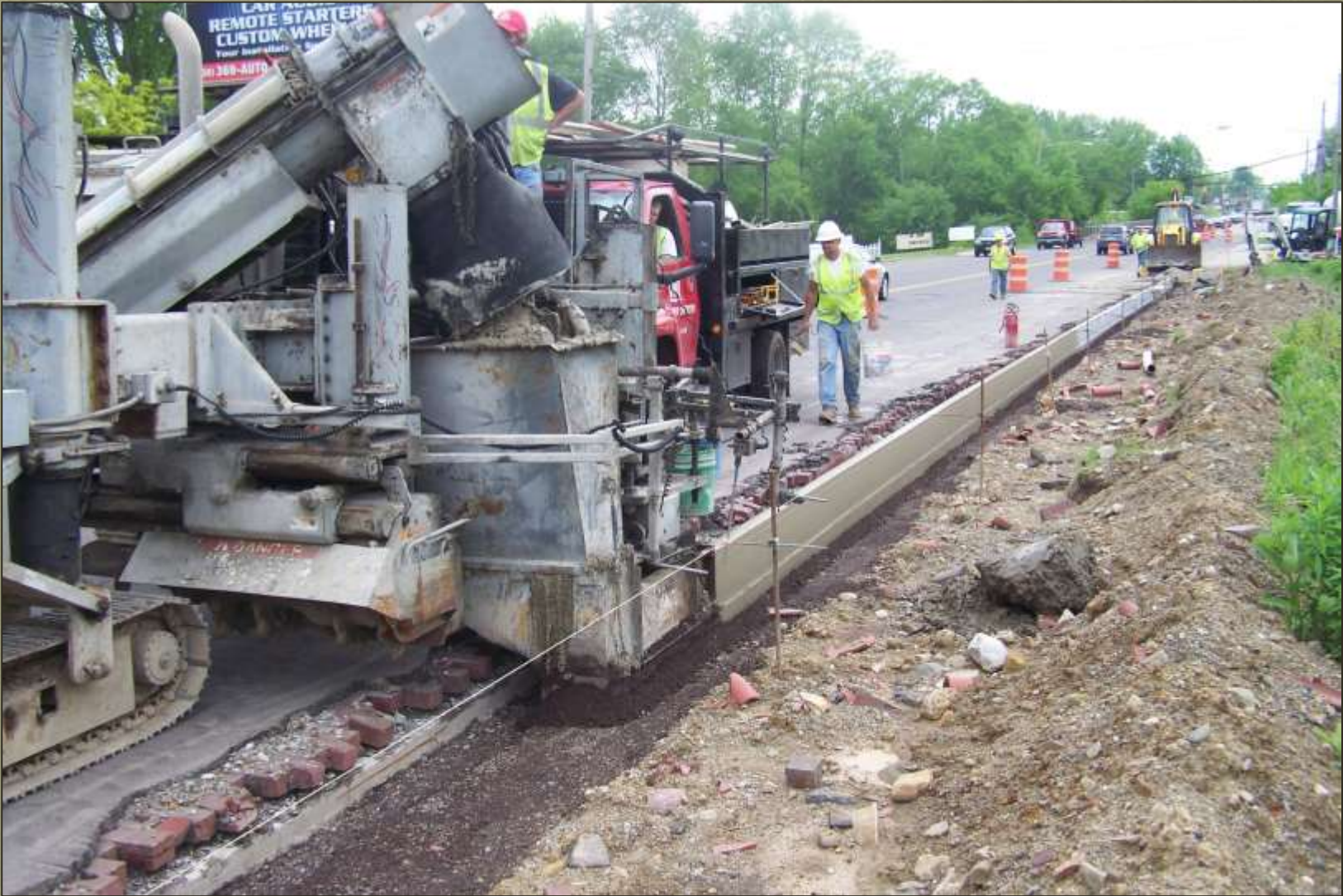
Parkman Road NW Phase 2 - 2011
