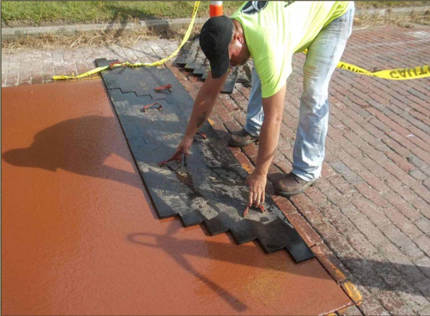
Brick Street Repairs – 2014 City Road Project Stamping pattern – September 10, 2014
