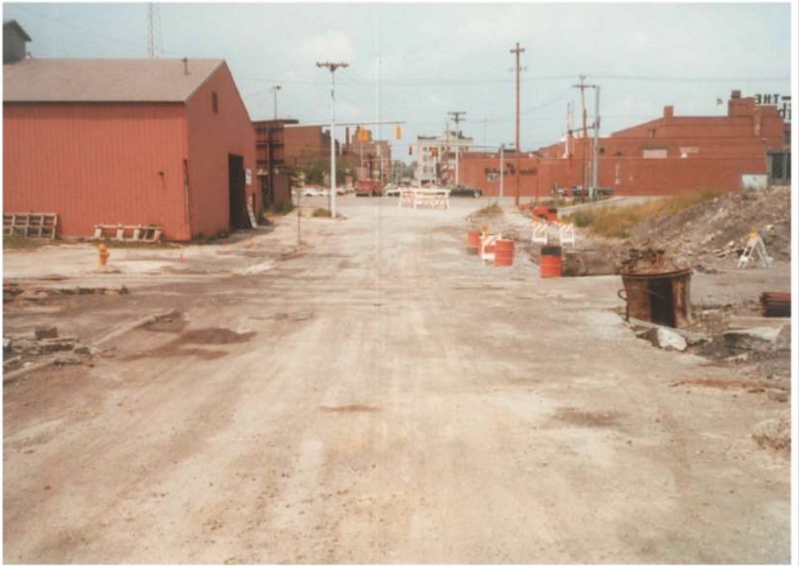
Pine Ave Widening & Storm - 1984
