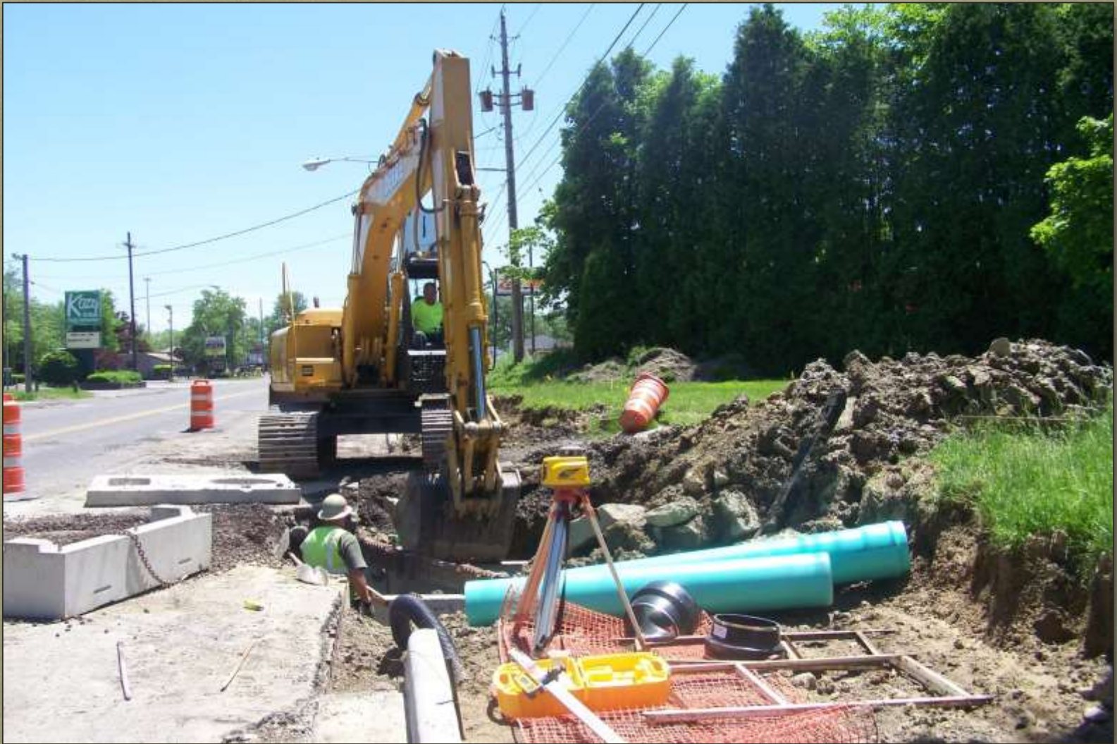
Parkman Road Phase 2 - 2011 Storm Sewer Installation
