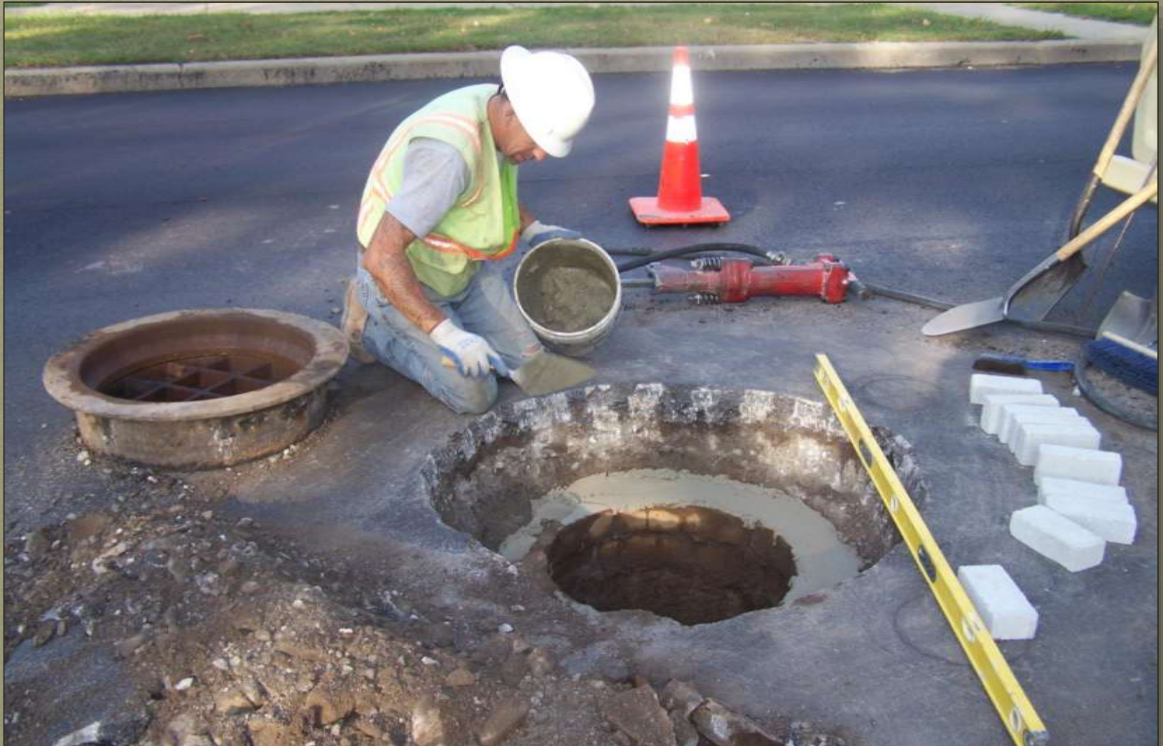
Mahoning Ave NW - 2010 Manhole Adjustments
