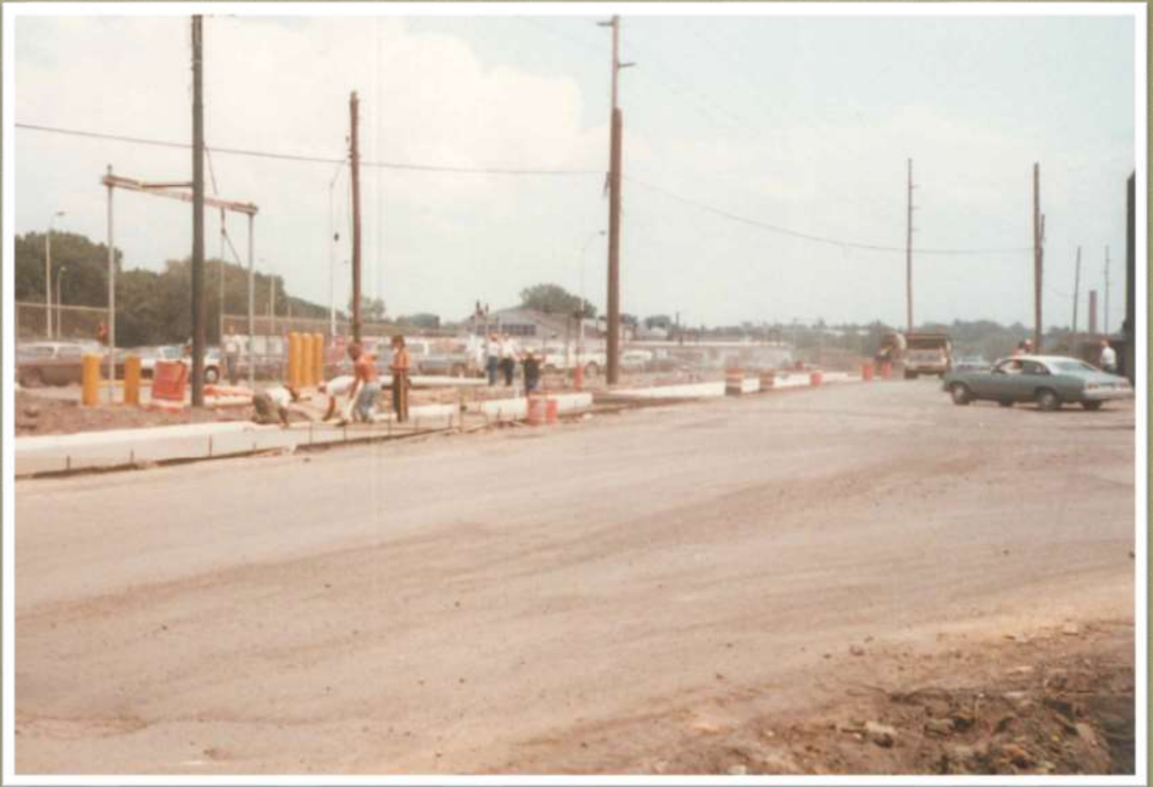
Pine Ave Widening & Storm - 1984
