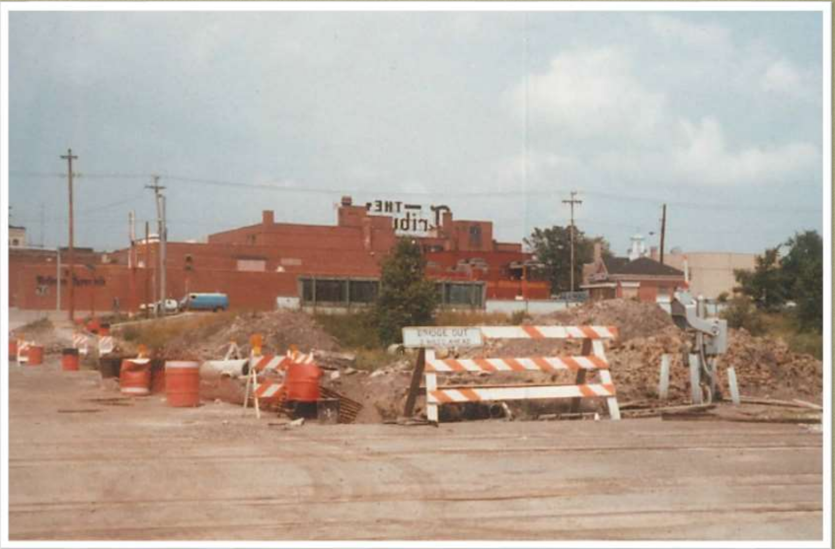
Pine Ave Widening & Storm - 1984
