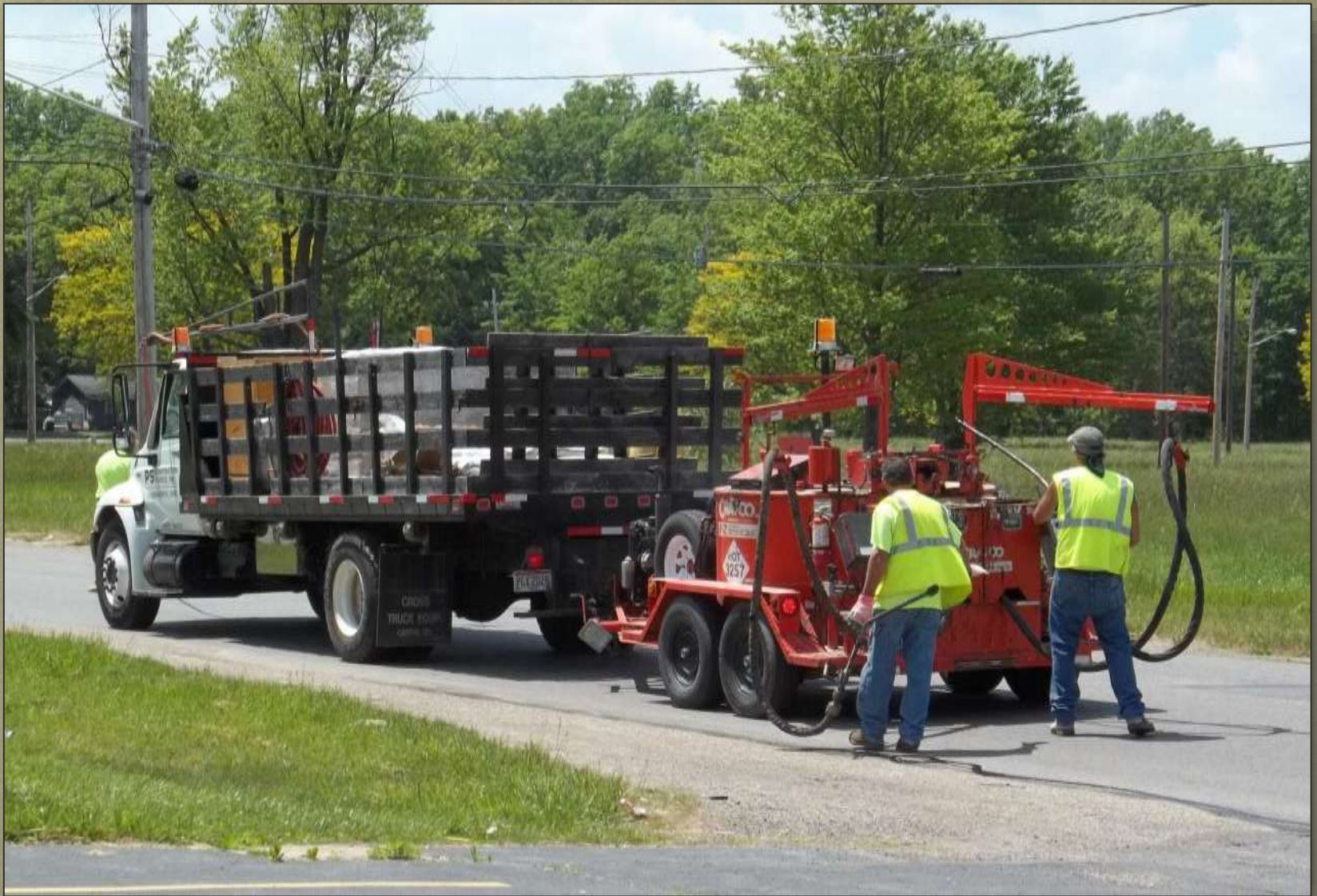
Crack Sealing on Nevada Ave SW - 2012
