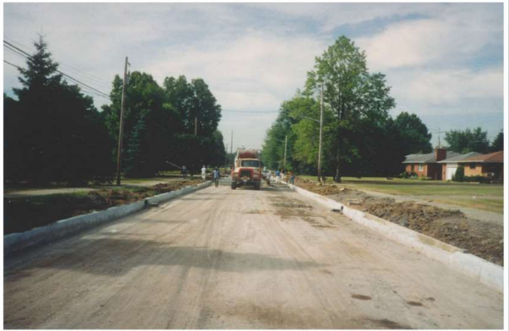
Tod Ave NW Reconstruction & Safety - 1993
