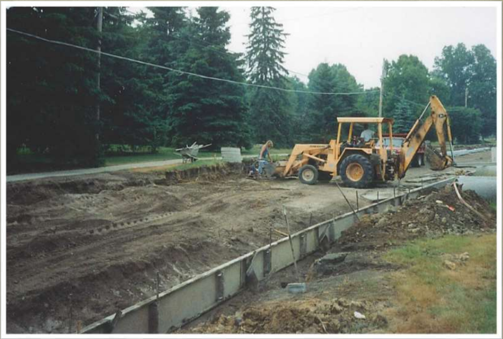
Tod Ave NW Reconstruction & Safety - 1993
