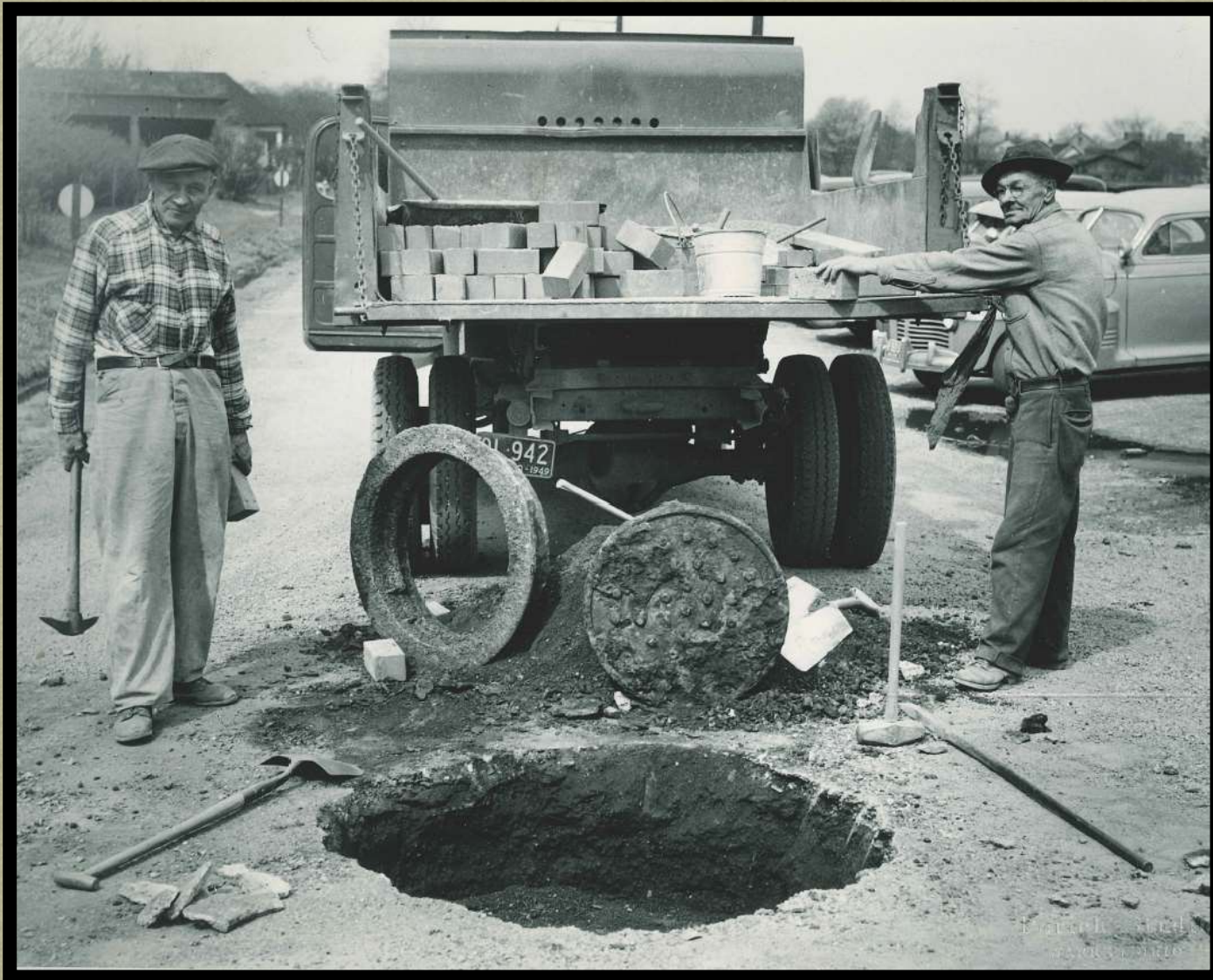
Fremont Ave NE Manhole Adjustments - 1949
