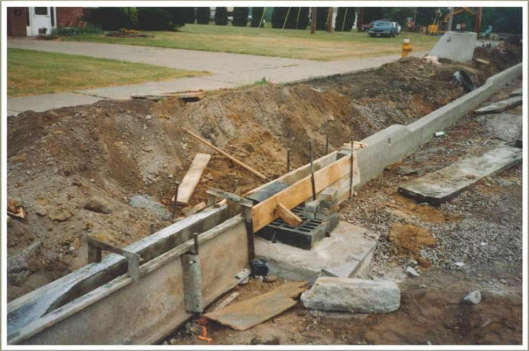
Tod Ave NW Reconstruction & Safety - 1993
