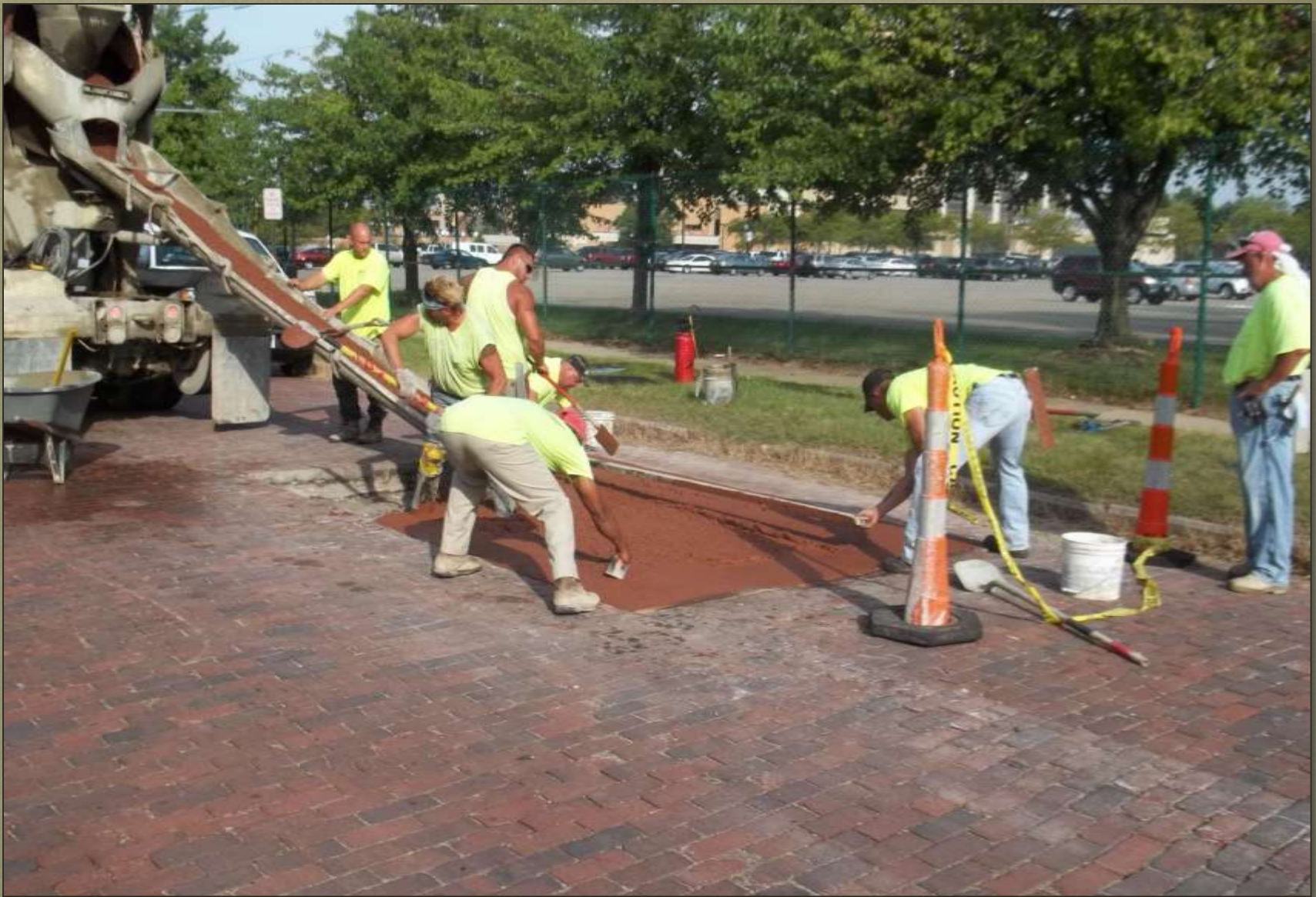
2014 City Roads Project - September 10, 2014 Brick Repair on South St SE
