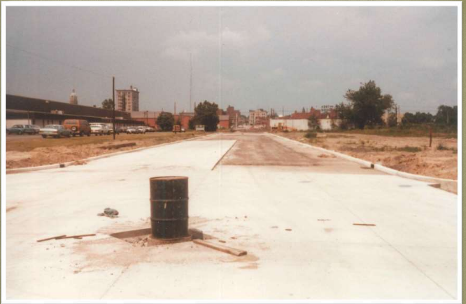
Pine Ave Widening & Storm - 1984
