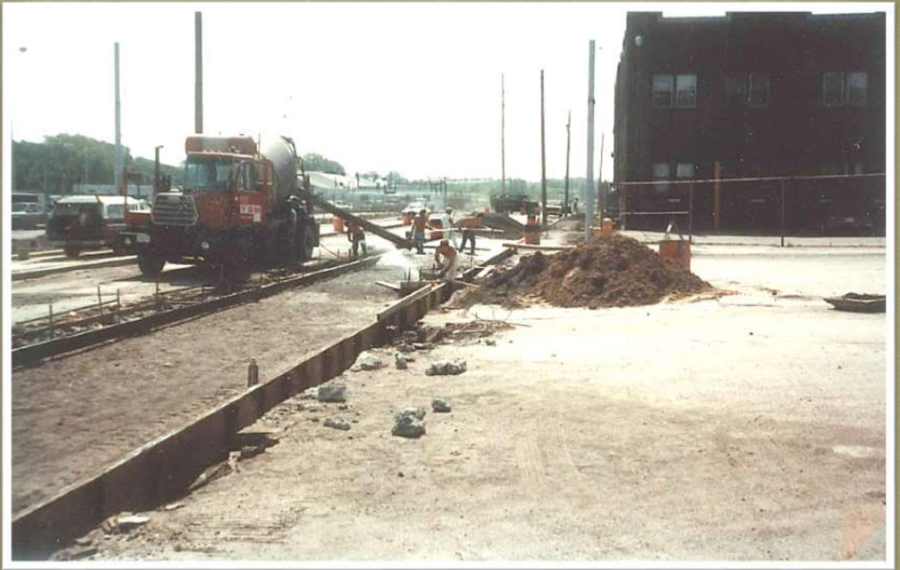
Pine Ave SE Widening & Storm Sewer - 1983
