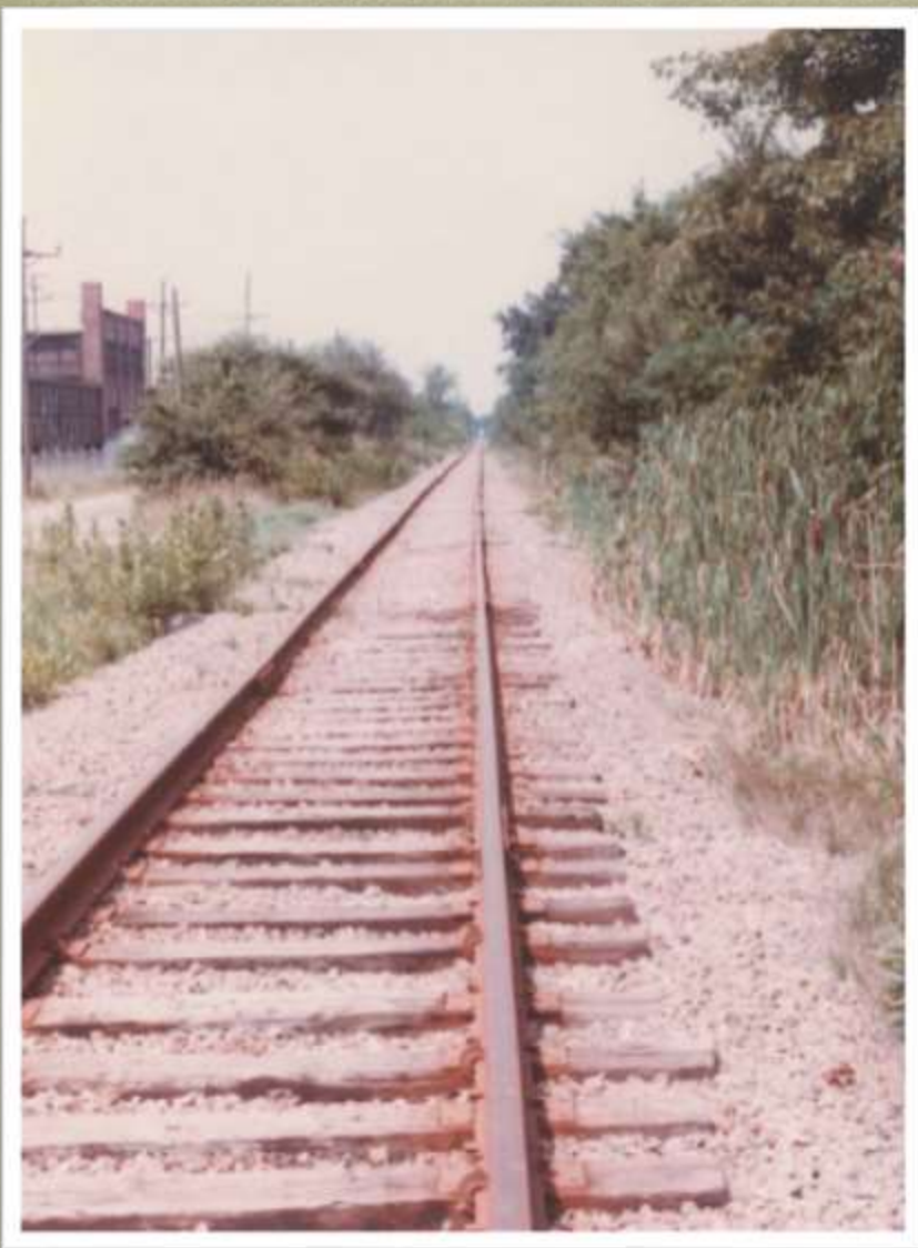
Railroad along Thomas Rd SE 1983
