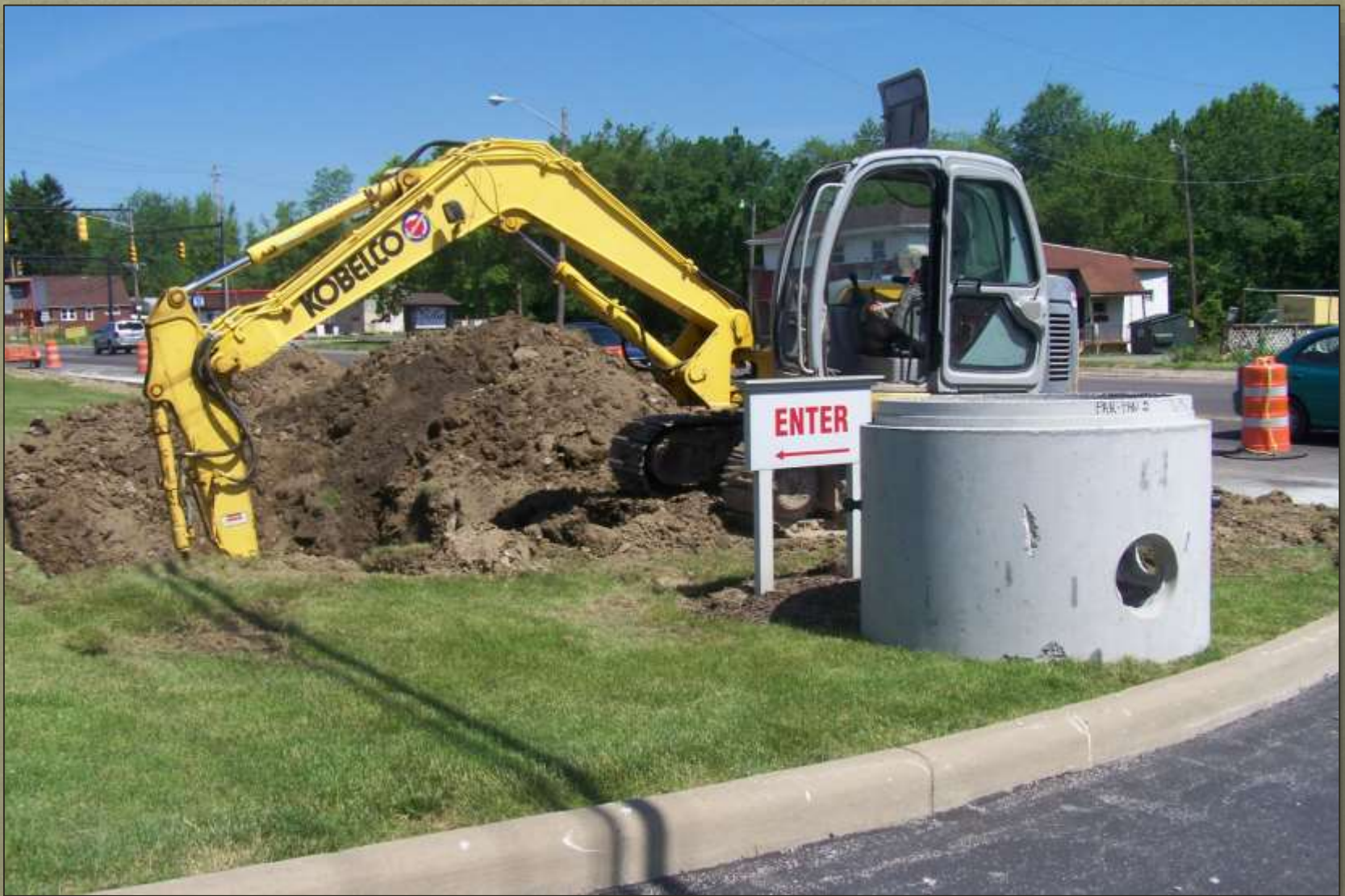
Parkman Road NW Phase 2 - 2011
