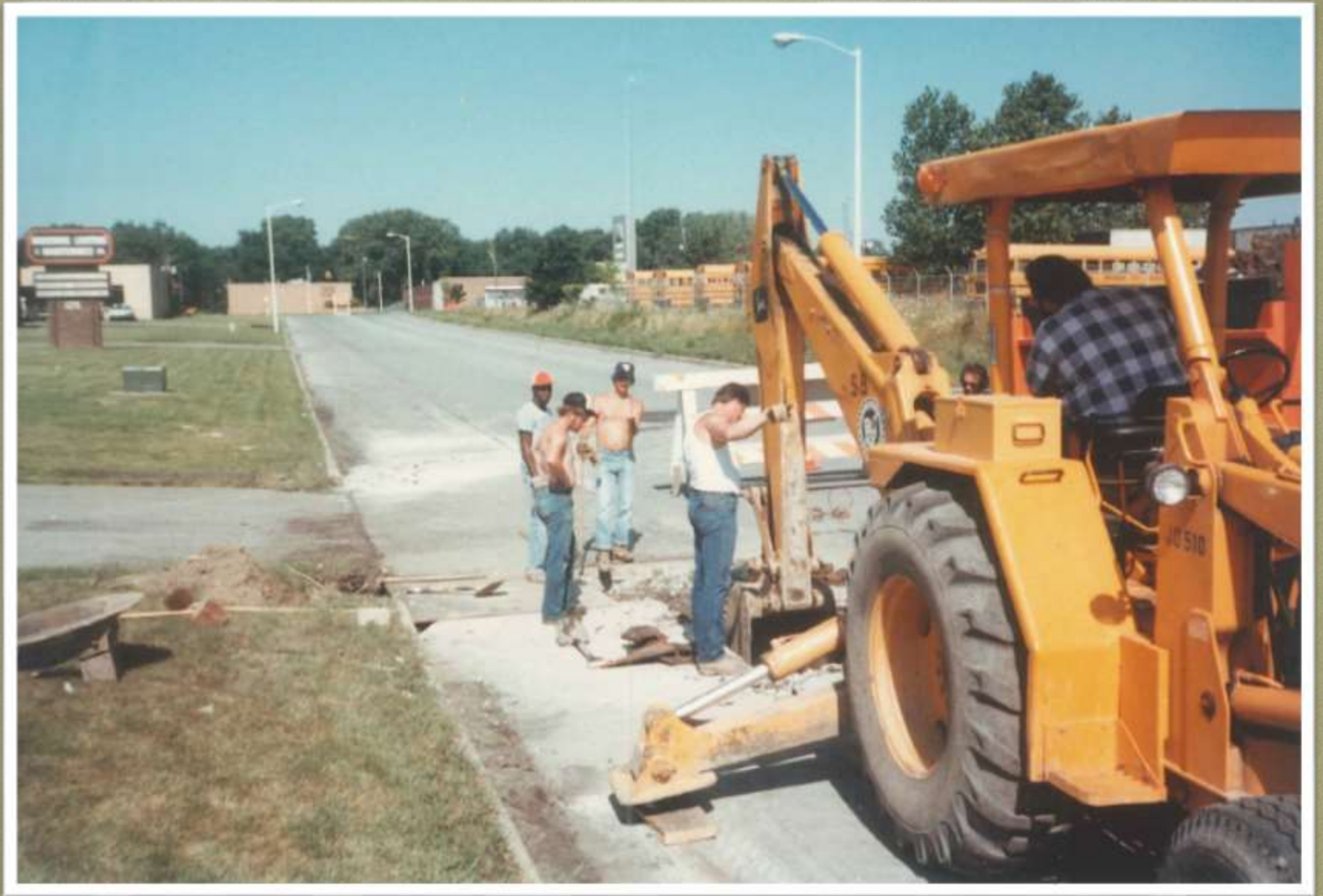
Pine Ave Widening & Storm - 1984
