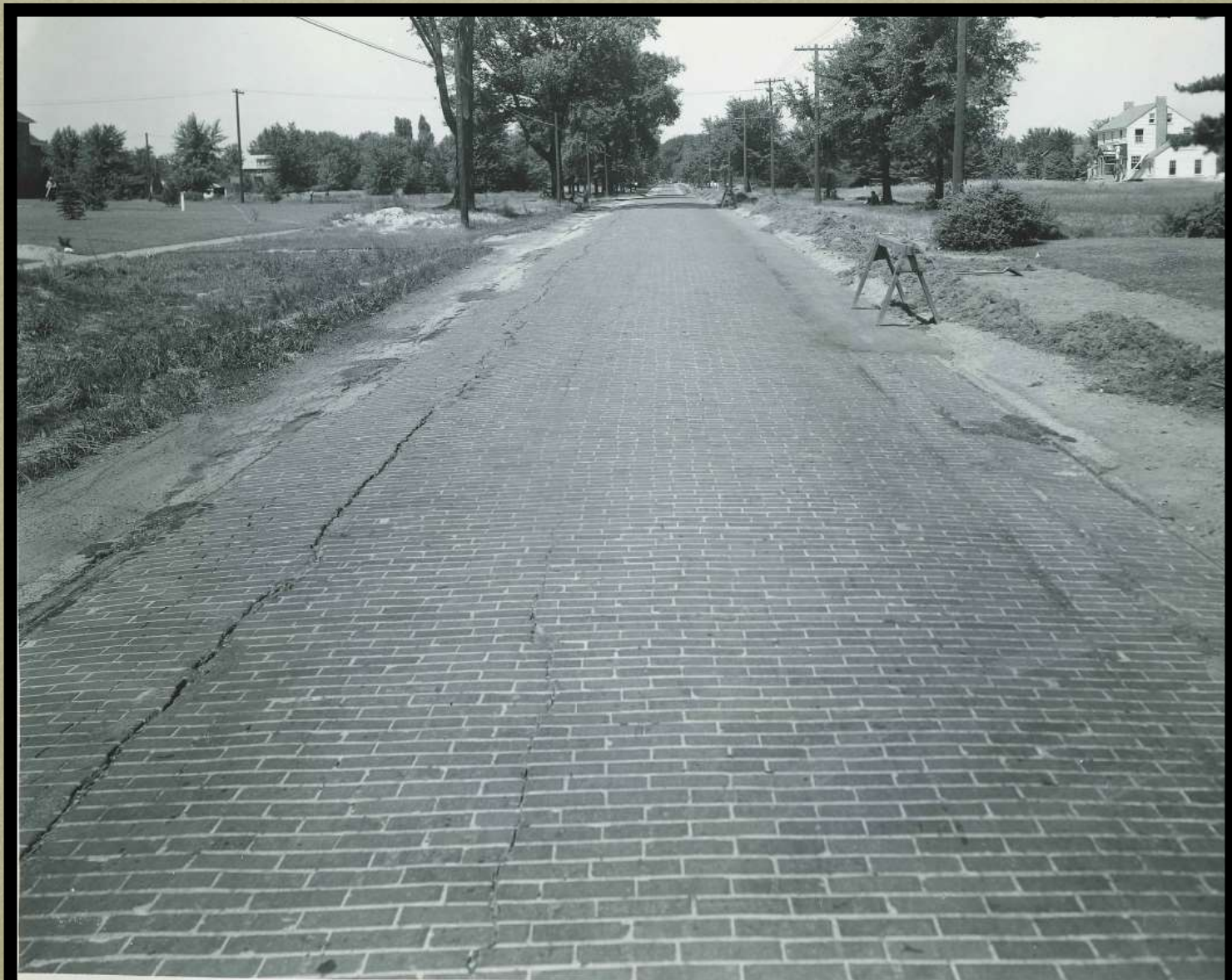
ON CENTER LINE OF EASTLAND AVE. LOOKING WEST
