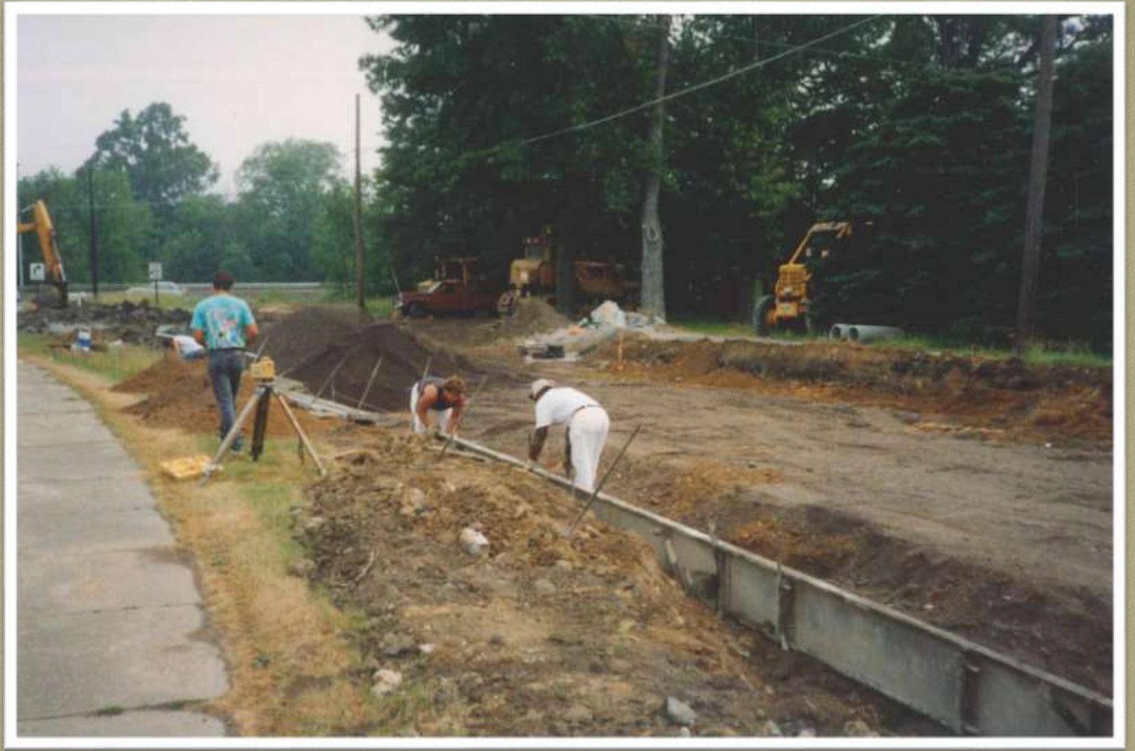
Tod Ave NW Reconstruction & Safety - 1993
